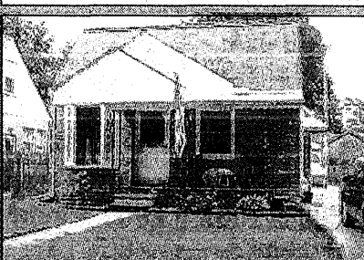
REDFORD $54,900 Well maintained and updated ranch with newer roof, windows, furnace, central air, kitchen and more! MLS 28145507 734-462-9800
