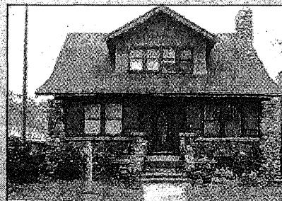
PONTIAC $129,900 4 bedroom, 3 bath home. Home features fieldstone fireplace in LR, formal dining room, and finished bsmt. Updated electrical & newer roof. Attached 2 car garage. MLS 27187624 248-673-2211
