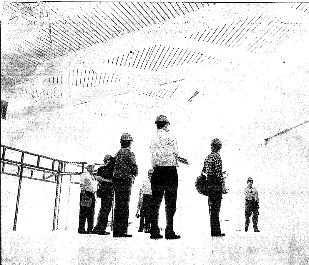
The new terminal's design isn't as flashy as the McNamara Terminal, but will be a major improvement over the aged Smith Terminal.
