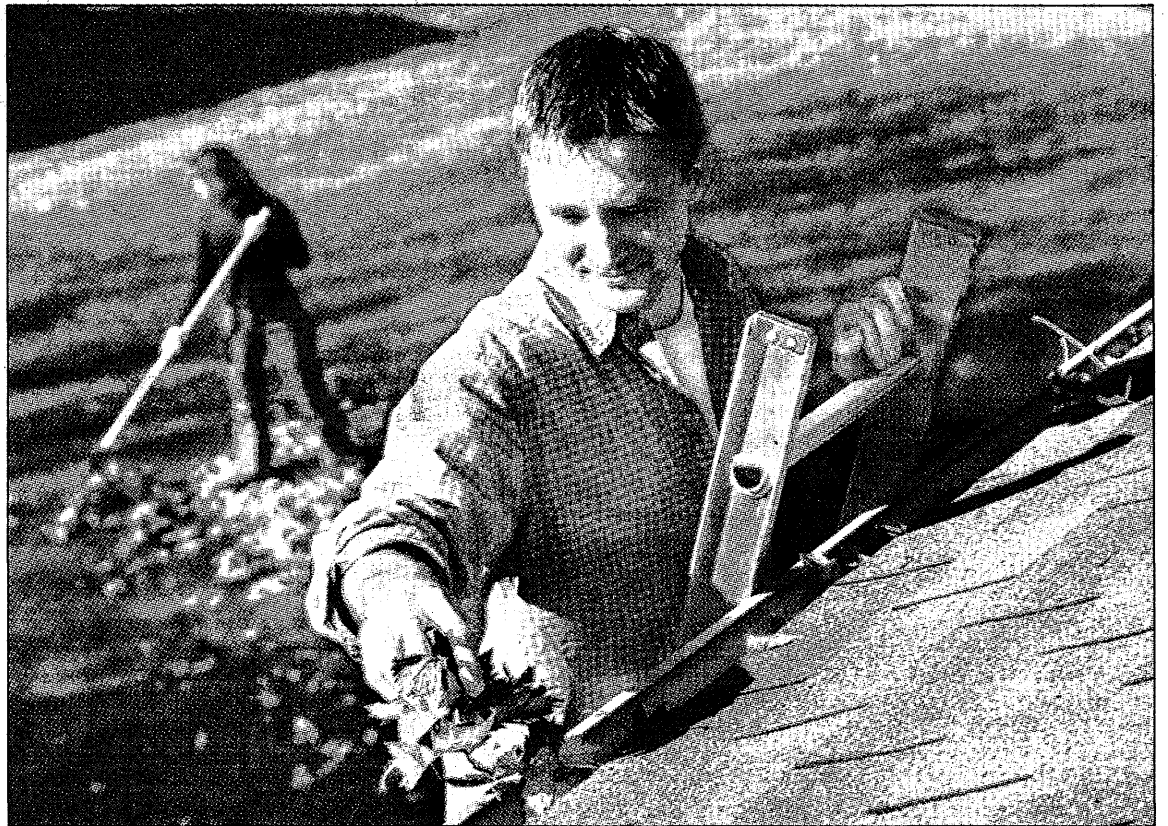
Cleaning out a winter's worth of debris from the gutters is an important part of inspecting a home each spring.
