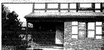
SOUTHFIELD $90,000 Completely remodeled 2 bedroom, 2 bath condo. New kitchen, new baths, new carpet, furnace and a/c. 107. Finished basement with lots of storage. Newer roof. MLS 27053324 734-462-9800
