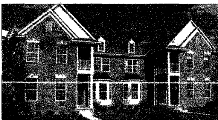
Georgetown-style condominiums feature floor plans with a main floor master suite, large lofts and private patios
