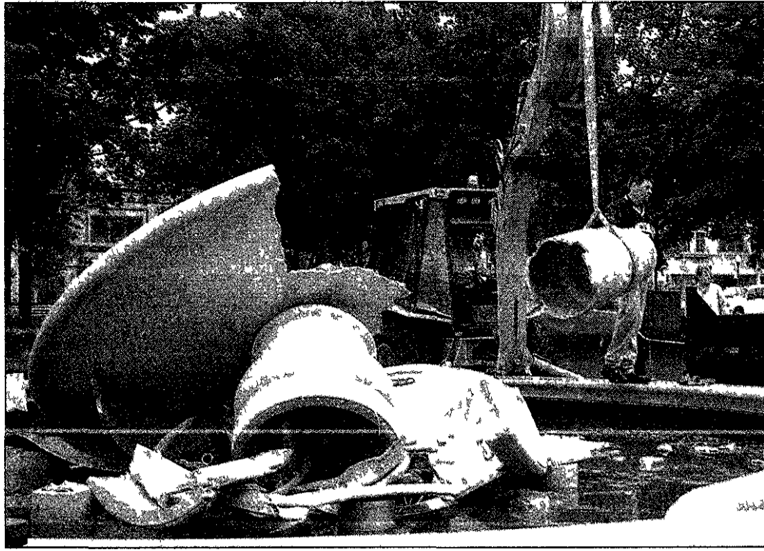
City officials are considering options for paying to replace the fountain in Kellogg Park which collapsed in May while contract crews were trying to stabilize it
