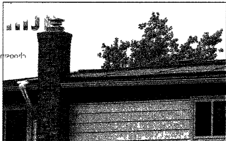
Solar collectors, mounted on the roof of the home of Kelly and Jason Kleinsorge, warm water inside the panels before the water re-enters the swimming pool
