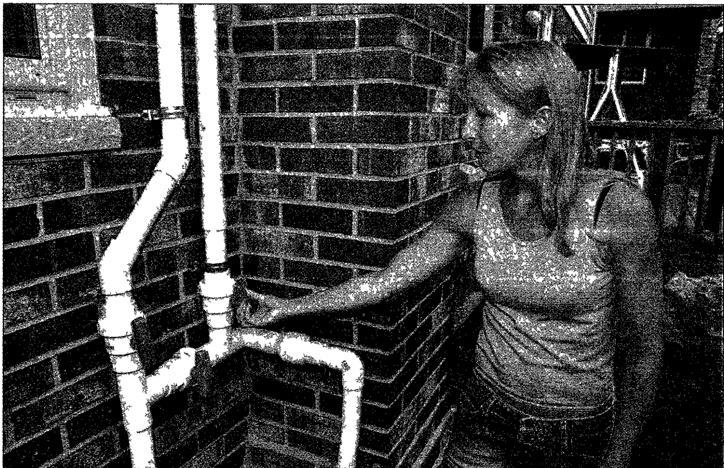
Kelly Kleinsorge keeps an eye on the sunshine and makes adjustments on the flow of warm water to the swimming pool at her home in Canton. The vertical pipes lead up to the solar collectors, mounted on the roof of the home.
