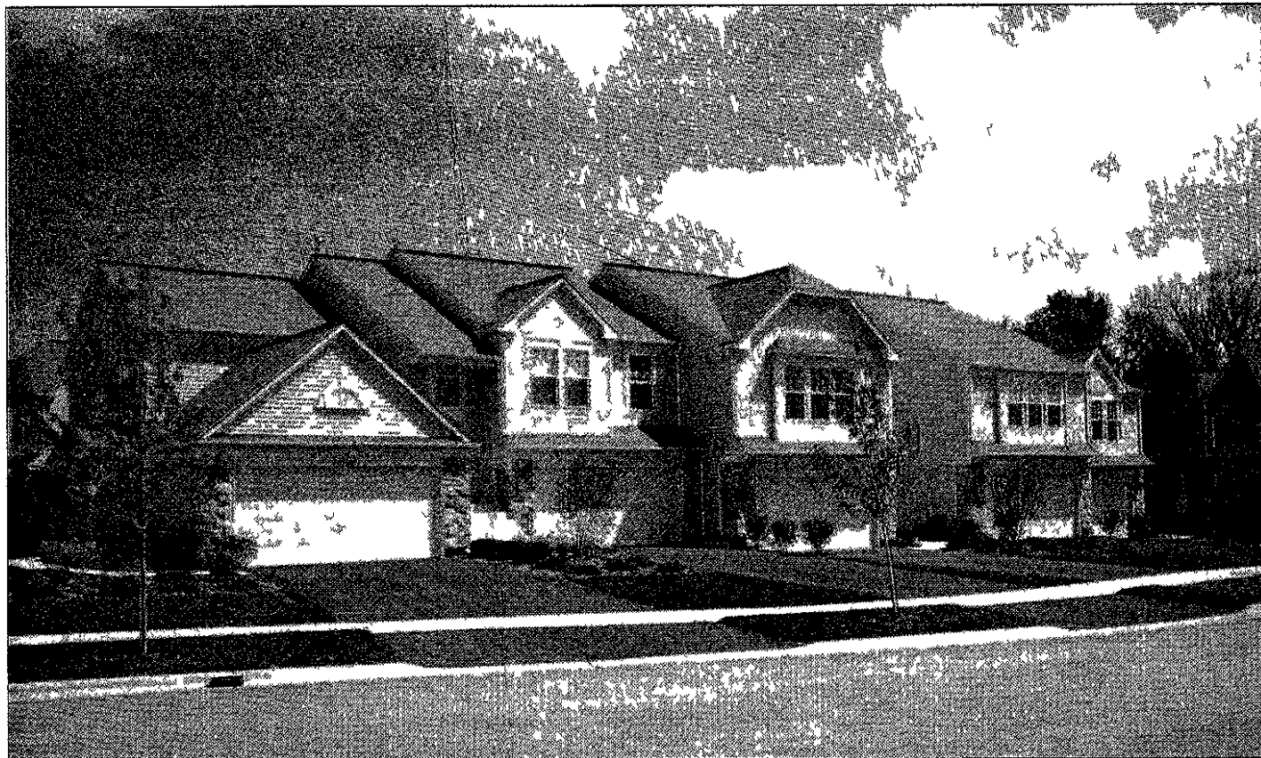
This rendering depicts what the front elevation of the two-story units looks like at The Villas of Riverside, but does not show all of the door front included in the final product.
