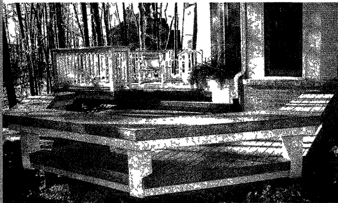
Above, the two risers between the two levels on this deck can provide extra space for seating At right screened-in porches are popular, according to Mike McCoy of Coy Construction The floor here is made of cedar
