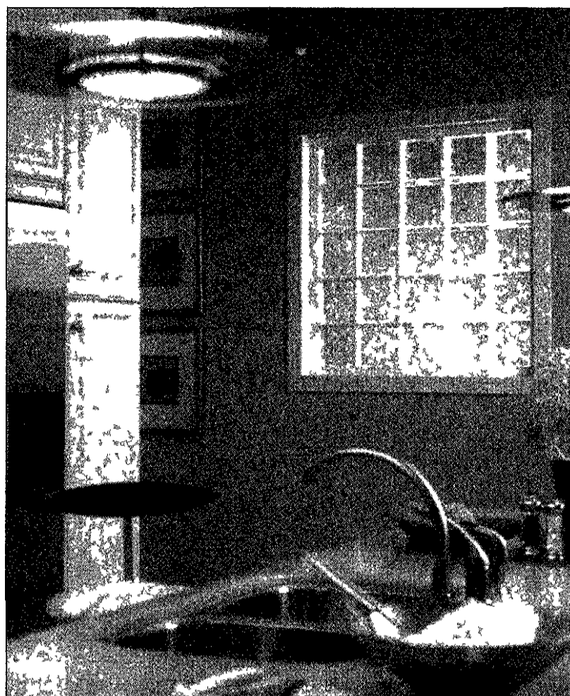
This prefabricated Hy-Lite glass block window allows light to flow into the kitchen while protecting the privacy of the homeowners.
