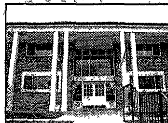
NORTHVILLE - Attention Flenters Great opportunity to live near the historic district Be the 1st to enjoy this updated starter condo Fresh paint newer carpet updated kitchen and bath Rent to own option $104 000 (25FAI) 248 349 5600
