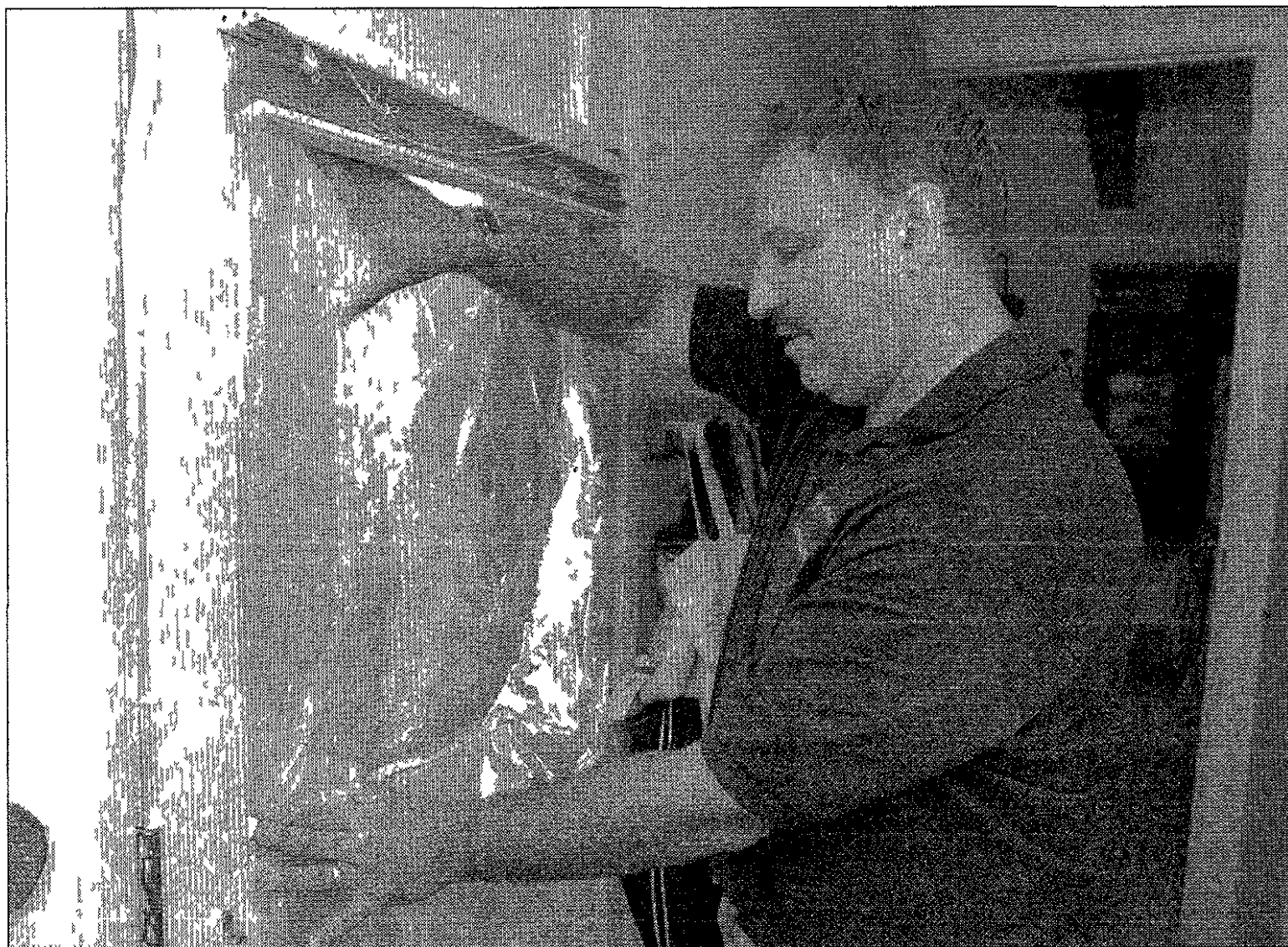
Larry Kaufman, DTE program manager and Observer & Eccentric energy columnist, places plastic sheeting over a door. Since the door does not have double-pane glass, the plastic will help cut the heat loss.
