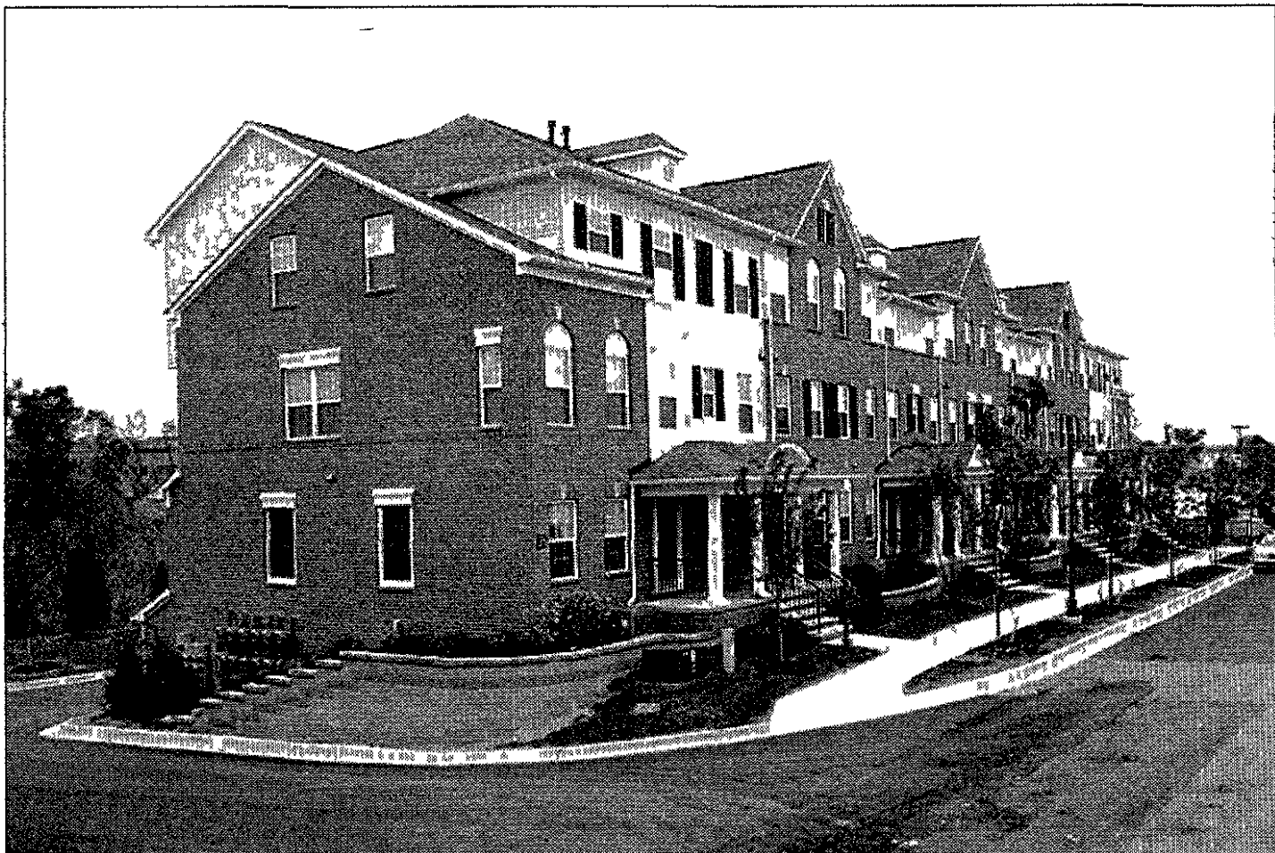
Several variations of luxury raised ranch and townhome apartments are available at Main Street Village.
