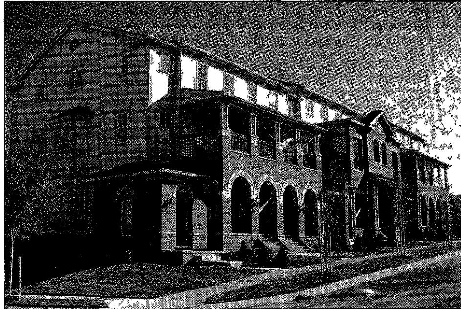
Condominiums with porches and balconies at Forester Square are placed close together near sidewalks and the street to foster interaction among residents.
