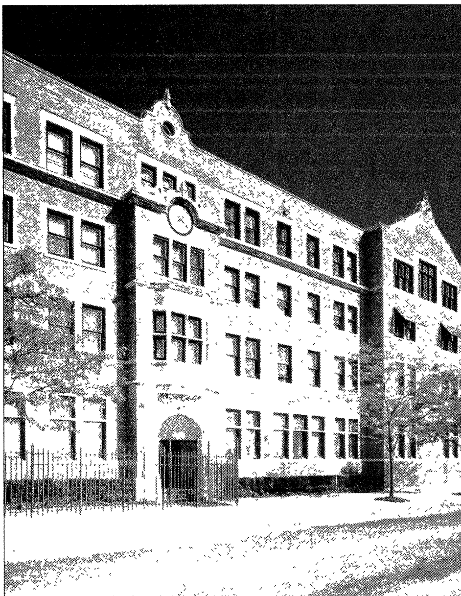
Apartments will be refurbished into condominiums at a historic warehouse on the edge of downtown Detroit.
