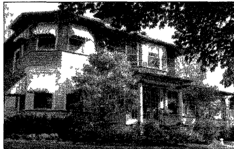
Among the six houses on the Plymouth Symphony League's holiday home tour is an almost 100-year-old Plymouth residence that is now a bed and breakfast inn. Holiday decorations, dubbed "A Victorian Christmas," feature a 9-foot Christmas tree in the old-fashioned front parlor.
