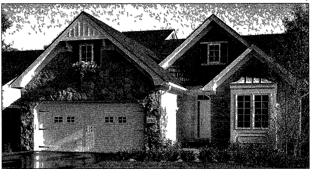
The building team at Hunters Grove maintains that many buyers prefer ranch-style condos with no steps.
