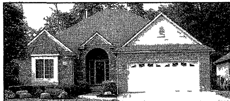
ALL HOMES HAVE A FULL BASEMENT & ATTACHED 2 CAR GARAGE
