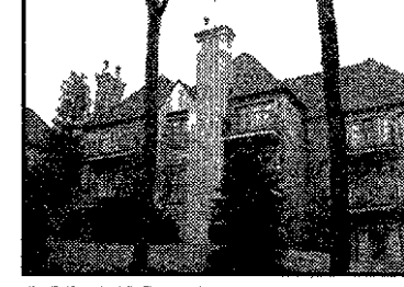
PICTURESQUE PINE KNOB SETTING Two story condo with finished walkout and two car garage will capture your heart The views and newer amenities are fault less $465 500 (35BRI) 248-363-1200
