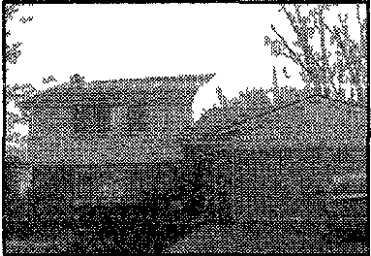
CANTON - Wooded lot with privacy! No neighbors behind so enjoy your privacy! Three bedroom 2 bath updated kitchen with oak cabinets new vinyl windows 3 doorwalls roof insulated garage door etc Family room with brick fireplace $219 900 (00RAI) 734 455 5600
