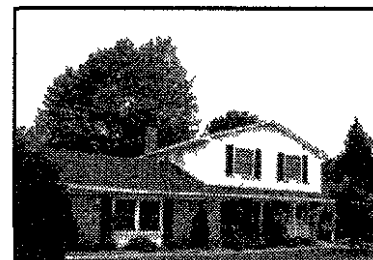
TROY Attention developers 3+ prime Rouge River frontage Splittable four cluster home gated community Four sewer tap rights Perfect for exclusive home community Includes existing home Mature trees $799 000 (99BEA) 248 524 1600
