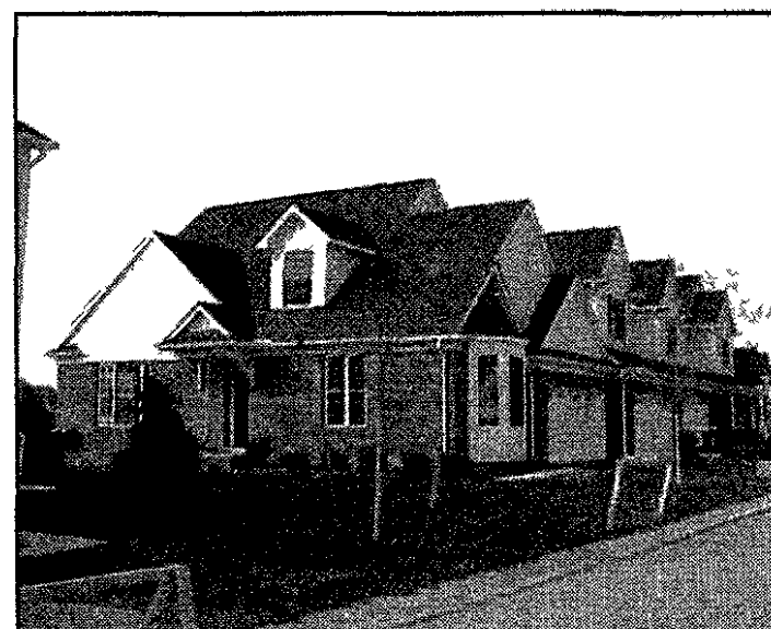
Garage orientation: In some buildings, the garage is oriented toward the main road; in others it's situated in back.
