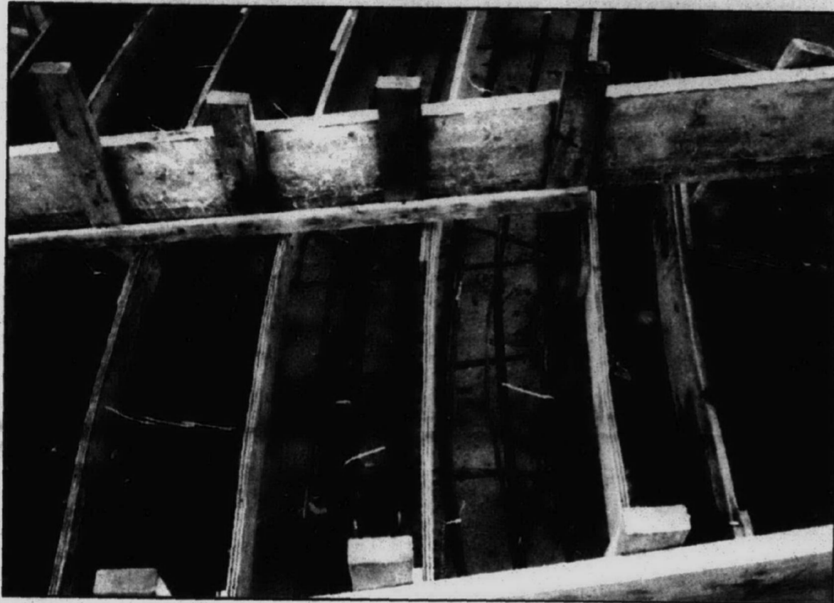
How it works: This is a photo taken by Snow Technologies Inc. of Livonia, which is building the new automatic snow and ice melters in the walkways and steps of the new Plymouth District Library. First the pipes are installed, followed by the cement.
