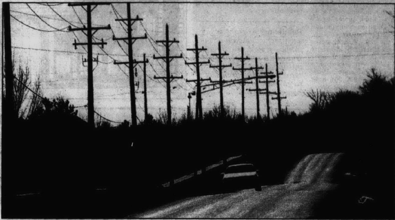
Paving: Ridge Road between Powell and Ann Arbor Road is unpaved, but the county has offered to help pay to pave the dusty roadway.
