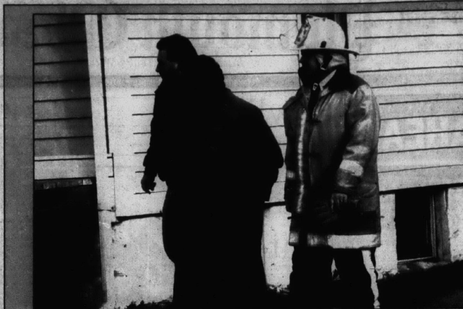
Undetermined: Arson is not suspected, but Plymouth fire officials are investigating the cause of a fire Wednesday at a four-unit apartment house. Fire chief Larry Groth escorts fire reconstruction staff Jim Peldo and Frank Bellomo with INRECON of Ann Arbor around the building pointing out areas they will have to board up.
