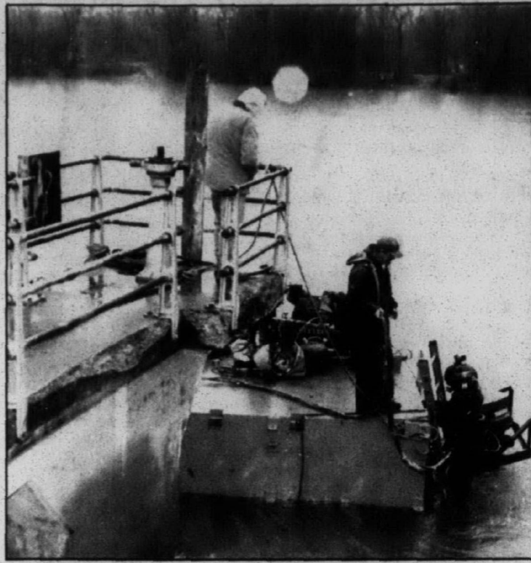
Diving right in: A diver prepares to enter Newburgh Lake to check for debris near a sluice gate and dam near Newburgh Road. A planned fish kill on the lake originally scheduled for this month was postponed until spring. The work is part of the lake's $10 million restoration project to excavate PCB sediments and eradicate fish that may contain those PCBs.
