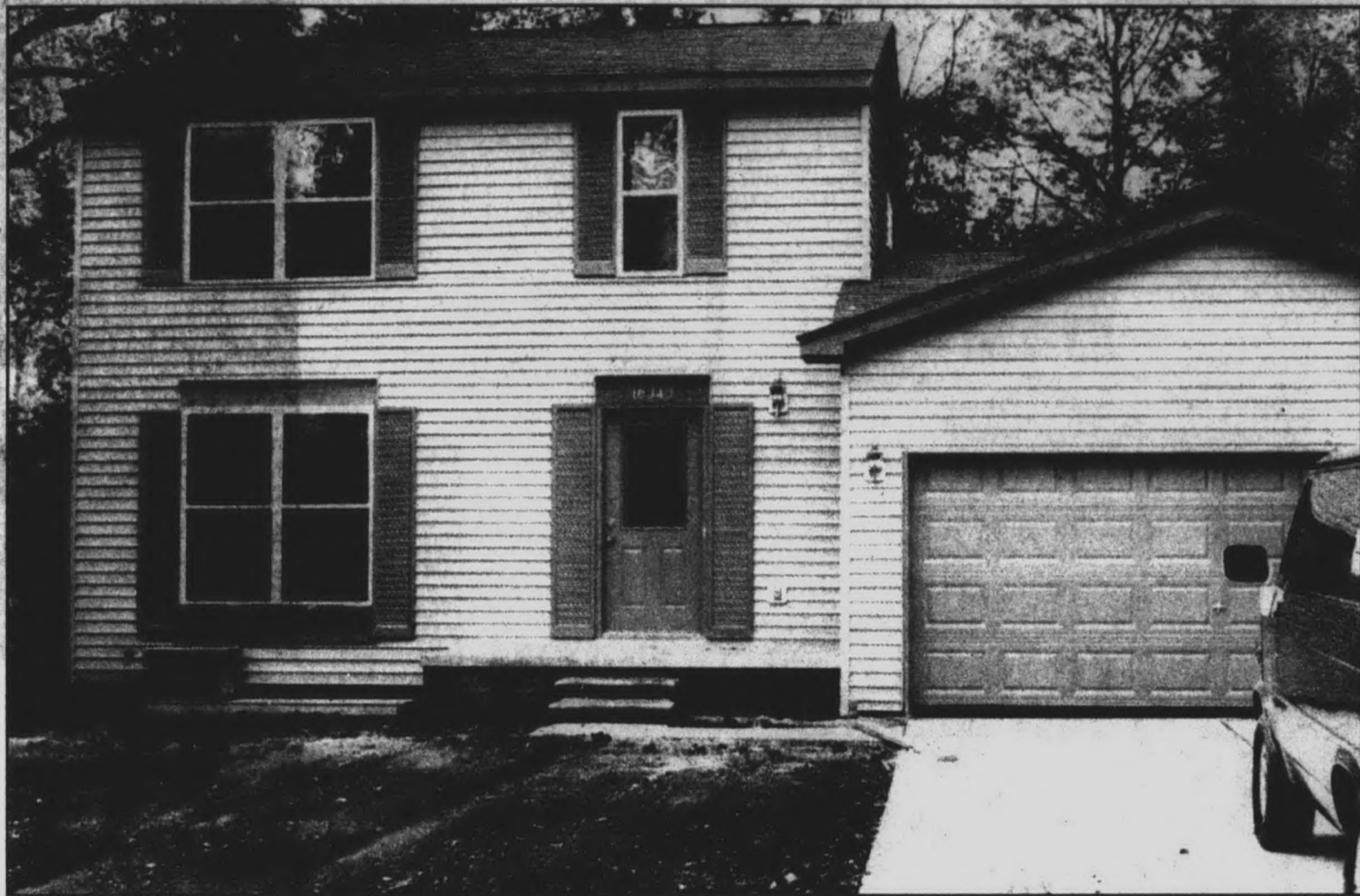
Meadow Downs: Builders at Meadow Downs can come up with a plan to suite any taste. But simple, functional designs like this are expected to be especially attractive.
