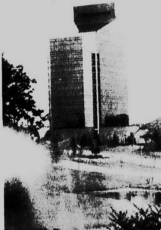
The Redstone-designed Grand Traverse Resort tower soars into the northern skies.
