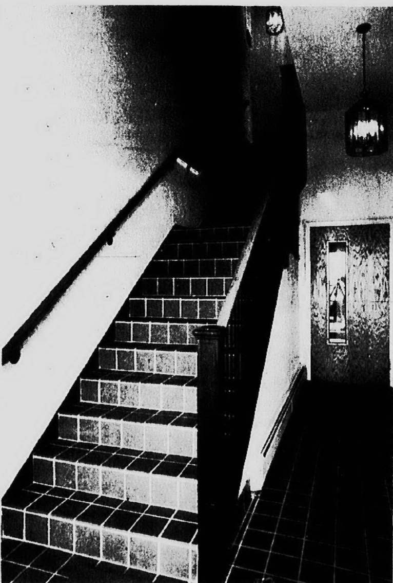
The entrance hallway and stairs have been completely redone.
