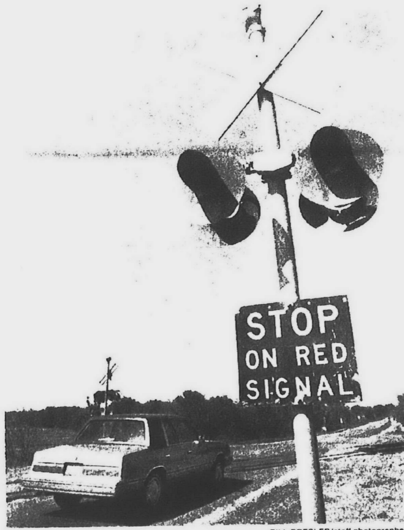
Plymouth Canton High senior David Knapp was seriously injured Saturday night when his car hit a train at this railroad crossing, Five Mile Road at Ridge Road. The train crosses the road at an angle. Plymouth police said the crossing signal appeared to have been operating.
