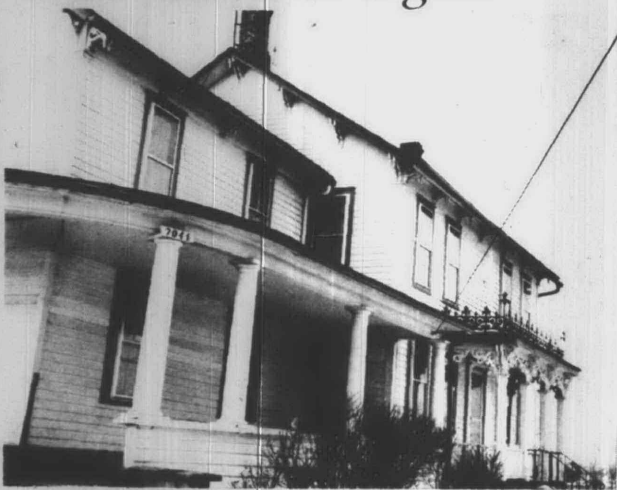
The small front porch shows the style of architecture popular when the house was first built. The wide sweeping veranda was added around 1900.
