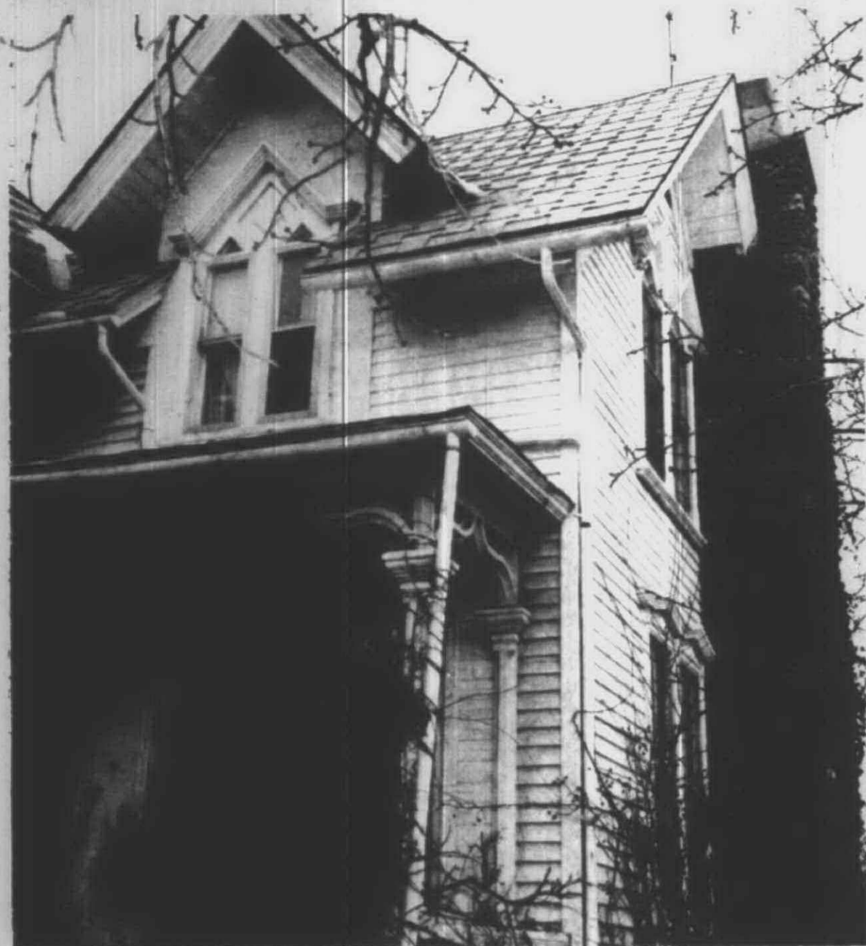
The house, with its pointed trim around the windows is an example of the Gothic revival style. Note the old chimney.
