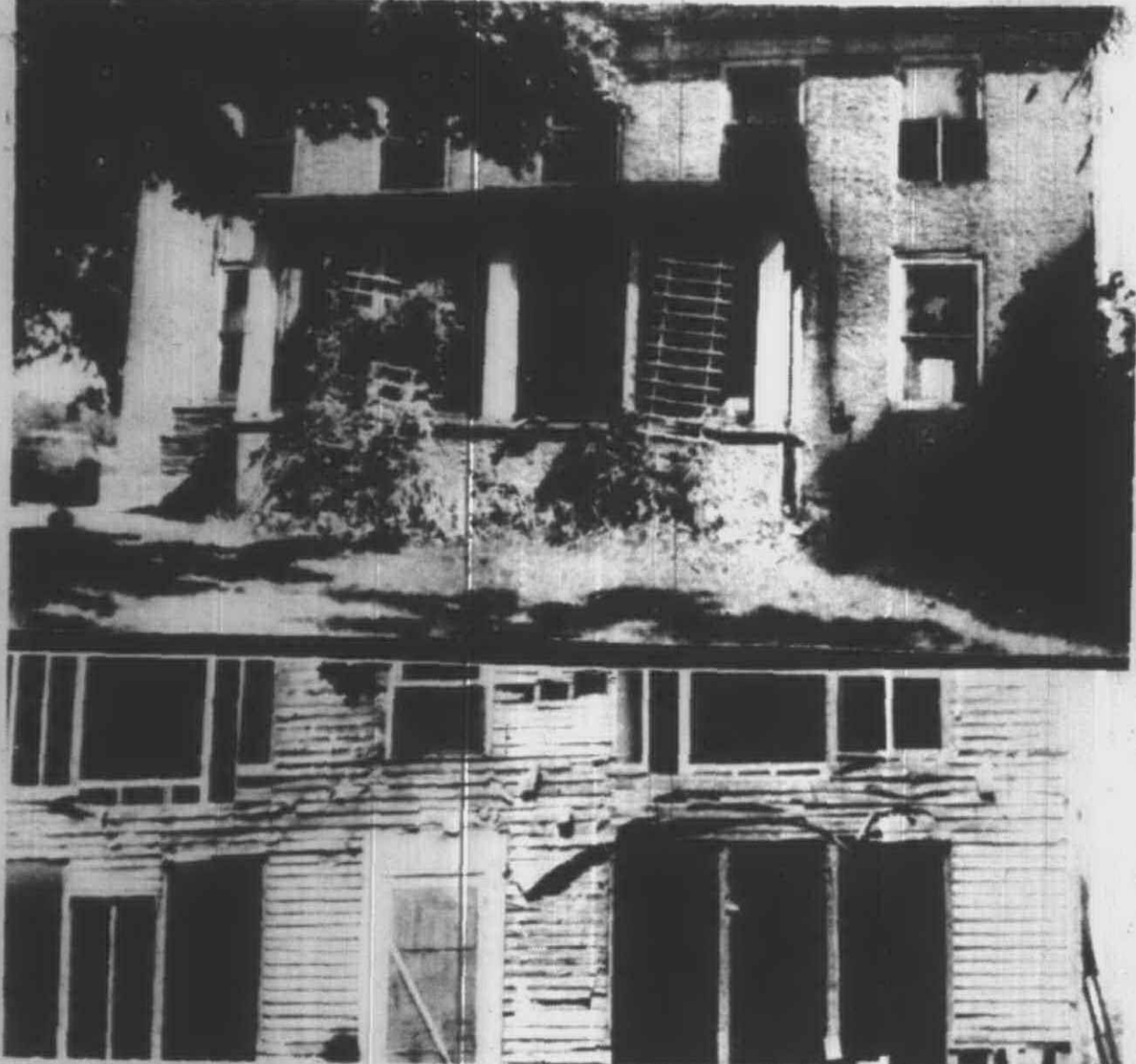
These pictures of the house, the top one taken when Froberg bought it, and the lower one as he was remodeling it, show the vast amount of work he did.
