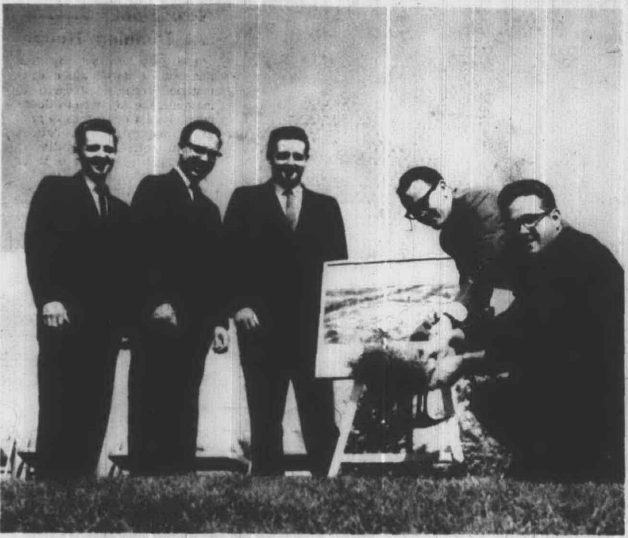
GROUND BREAKING ceremonies were held at the Plymouth Church of the Nazarene Sunday. From left, church officials Gilbert Wasalaski, Harold Anderson, Dean Hamlin, Pastor Ronald Moss and Russ Park toss the first spadeful of dirt.
