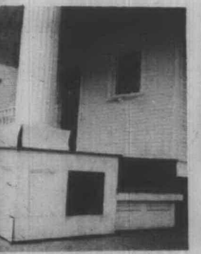
A remnant of bygone days are these high stairs which one stepped onto from a carriage.
