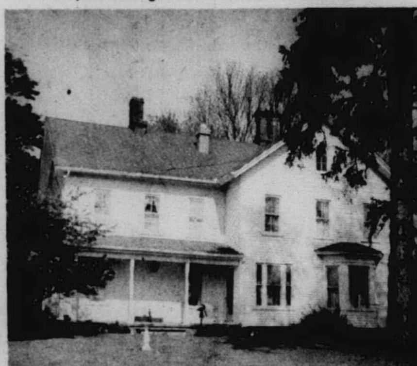
After — The front porch and pillars were added to the original structure, and the house was sided with aluminum. The only painting that must be done to the exterior is the pillars on the porch.
