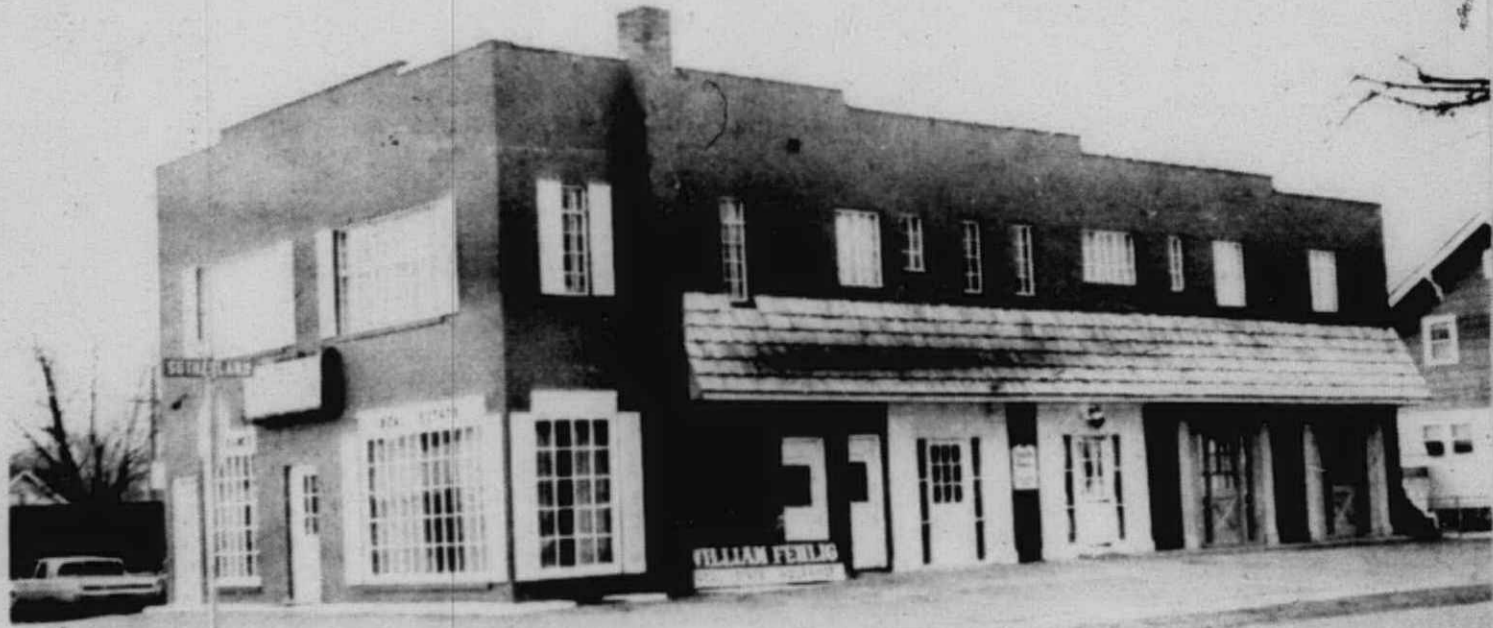
THE COLONIAL TOUCH shows itself on William Fehlig's new real estate headquarters office building. Presently Fehlig and Loren C. Gould's Gould Homes, Inc. are in the building. And Fehlig hopes to have three other office suites rented soon.
