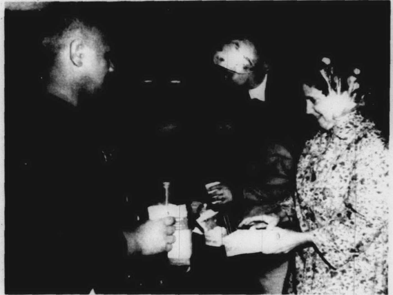
RAIN AND FOG made the job of capping a gas well near Sheldon Road tough last Wednesday night, and Plymouth Township firemen were called in to lend a hand. Ernest Honke, of the Plymouth Township fire department, was one of many treated to coffee and hamburgers by the Powderpuff's, the firemen's wives.
