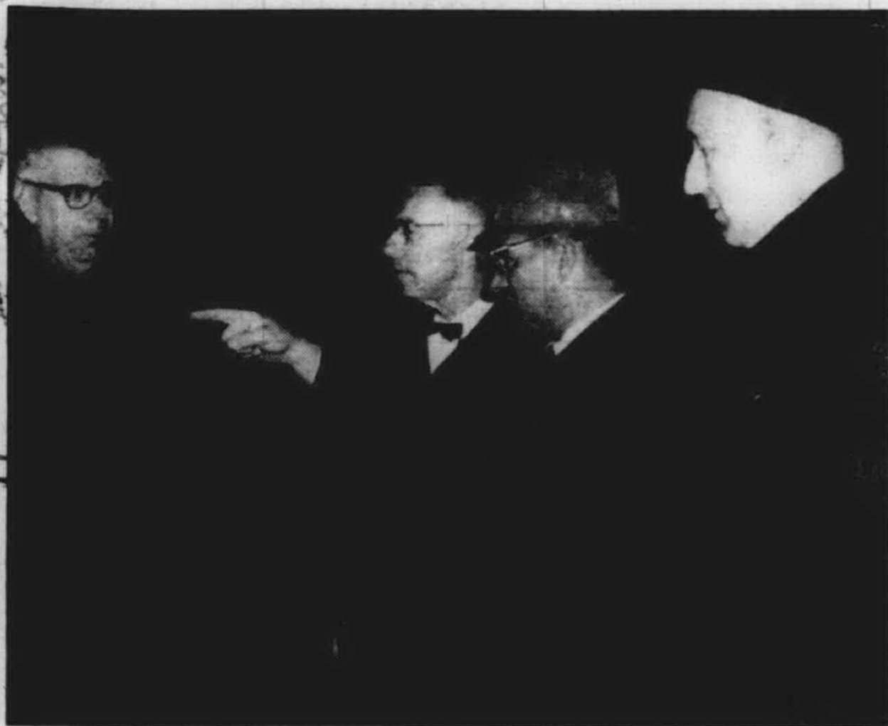
INSPECTING THE INSIDE of the old reservoir, located at the end of Reservoir Rd., off Edward Hines Dr., Saturday morning were, left to right, Acting City Manager Kenneth Fisher, City Commissioner James Houk, Department of Public Works Superintendent Joseph Bida and Mayor Richard Wernette. The men were looking at the reservoir, drained of water, to determine if it were worth patching and using.
