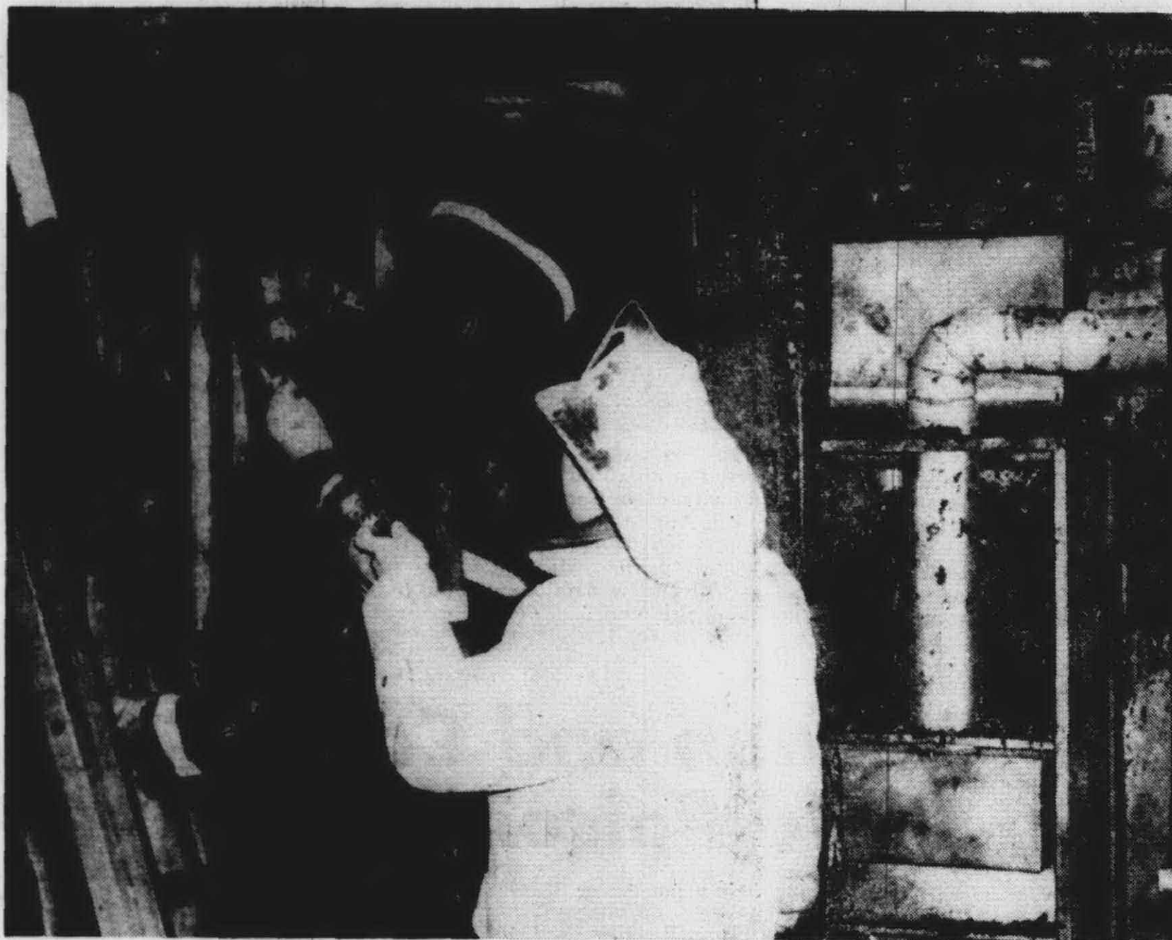
A CLUBHOUSE at Crestwood Apartments suffered extensive damage as a result of a fire early Monday night that started in a furnace compartment and spread to nearby walls and ceiling. Firemen had the blaze doused in minutes. An
