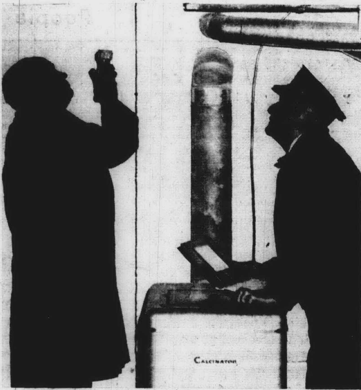
BUILDING inspector Charles Thompson (left) and City Assistant Fire Chief George Schoeneman inspect a basement of a Crestwood apartment unit to see if recommended changes have been made since a Feb. 21 fire in which an overheated incinerator like the one shown here started a fire that shot through an inside wall and mushroomed in a second story apartment. The City had asked that the pipes on the incinerator be fastened better and that certain fire stops be installed in the recently constructed buildings. The pipes were fixed but the latest inspection revealed a need for more fire stops. In the photo below, the arrow points to a hole where fire officials fear fire might spread from room to room. Immediately to the left is a hole for wiring that also needs fire stopping materials plugged into it. Thompson said the owners would be notified of the violation and given time to fix it. The inspections are part of a stepped up fire hazard check in all city multiple dwellings that had been urged by Commission Arch Vallier at a recent City Commission meeting. Both Thompson and Schoeneman issued a statement to apartment owners, telling them to expect a full inspection of their units in the near future. The Feb. 21 fire was the first of two recent fires at Crestwood units. (See story, Page One).
