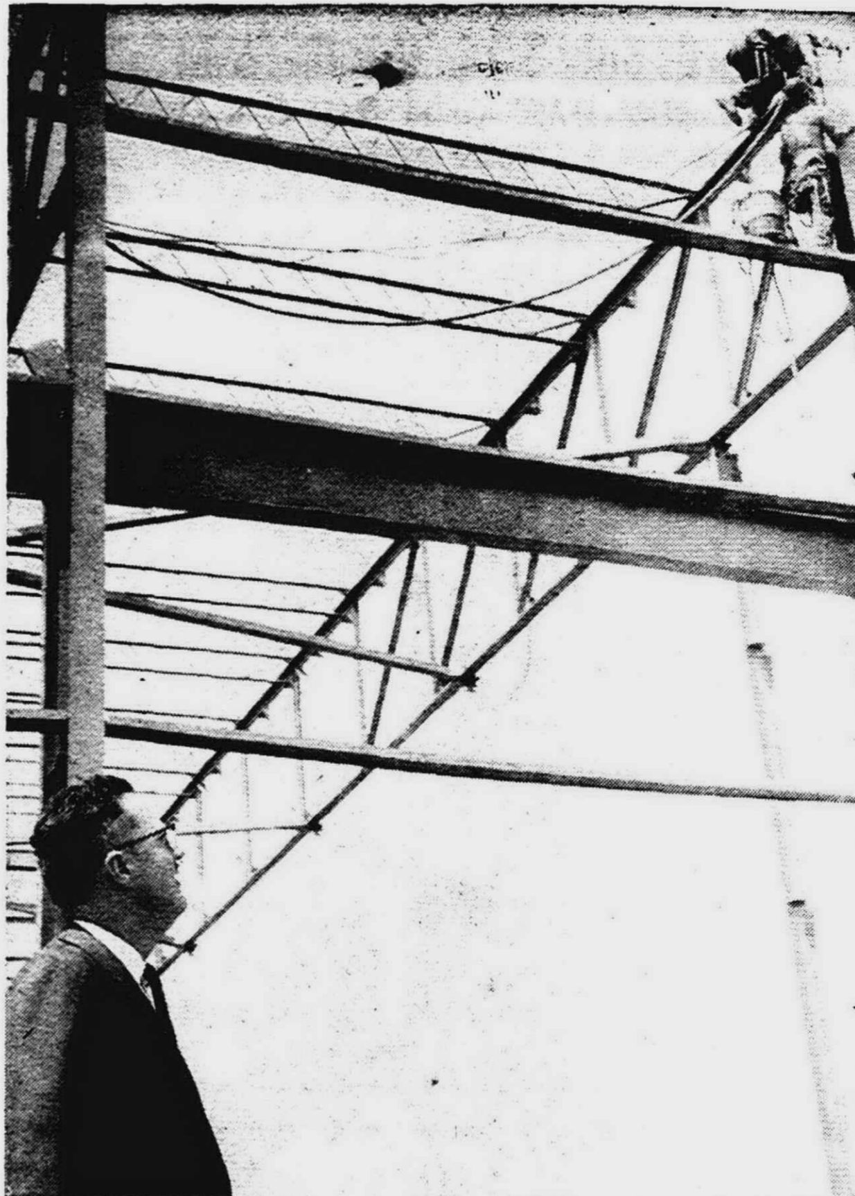
WORK WAS WELL along last week on the $1.5 million addition to Evans Products Company's Plymouth Township plant as workmen had nearly all of the structural steel for the 60,000 square-foot addition in place. John P. Moorhead, Northville, Evans director of engineering, watched a pair of workers Monday as they clambered, high up on the steel framework of the building. The building will house production facilities for Evans' DF-C coil railroad car. It is scheduled for completion early this fall.
