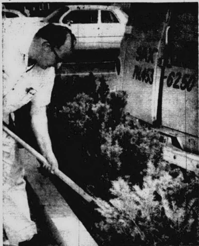
THE FINAL touch for the parking lot between the new First Federal building and The Plymouth Mail was the planting last week of shrubs in a small space at one corner of the parking area. Harley Smith, of Saxtons, is shown putting the shrubs in place.
