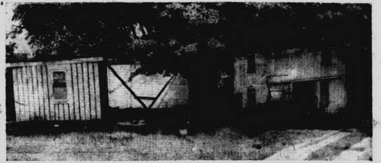
A PLYMOUTH LANDMARK , the old carriage house on the former Hough property, 243 N. Main, will be put to new use soon. Bought recently by Harold E. Guenther, 1142 N. Holbrook, it will be moved to the rear of the Guenther home and used to store a 1917 LaFollette fire engine and a 1928 Packard owned by Guenther. The Guenther's have long been interested in the heritage of Plymouth and Mrs. Guenther said if they had the money they would restore every old house in Plymouth.
