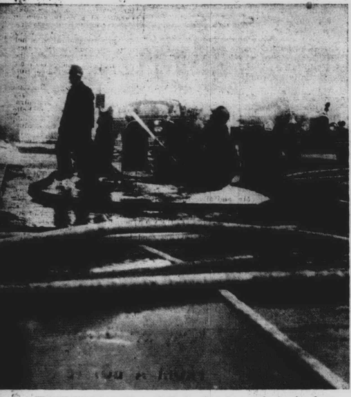
CROUCHING to get beneath the low-hanging smoke issuing from the burning building, firemen direct a fire hose into the flames. Total water used in battling the blaze is not yet known, but at one time there were seven 2 1/2-inch hoses in use, each issuing 325 gallons of water per minute. The rubble of the building continued to smoke Monday night and much of Tuesday. However, there were no cases of firemen suffering from excess smoke inhalation and there were no injuries.
