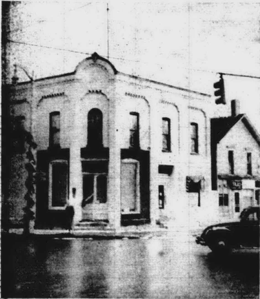
THE CORNER barbershop locked its doors forever last Saturday. Owned by four proprietors since 1902, the shop and adjacent buildings will be torn down soon.
