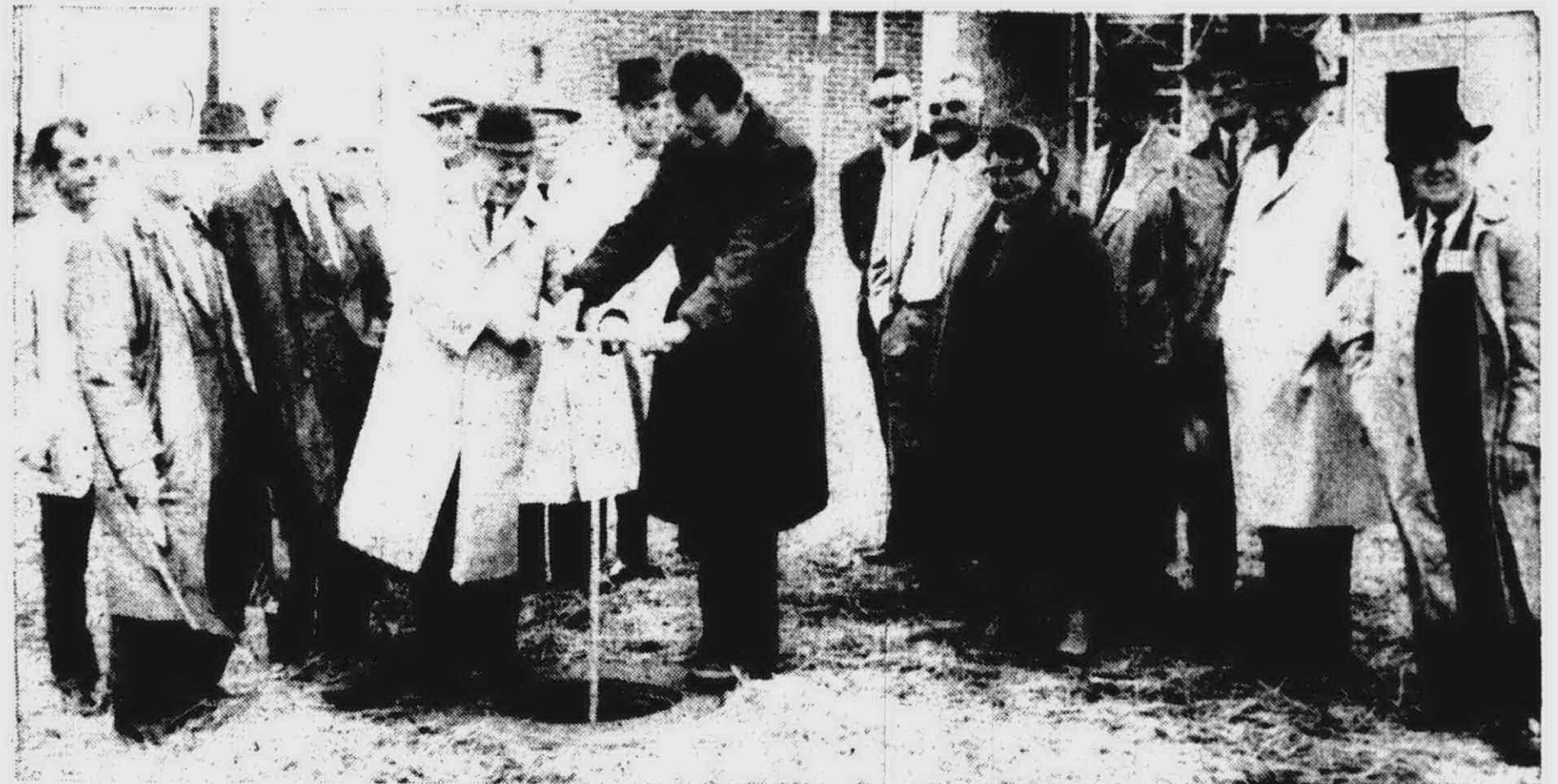
LET HER COME! Detroit water is now flowing in Plymouth Township mains and a ceremony to officially hail the new system was held last Friday noon. Township, Wayne County and Detroit officials, as well the contractor and engineers were on hand as Gerald
