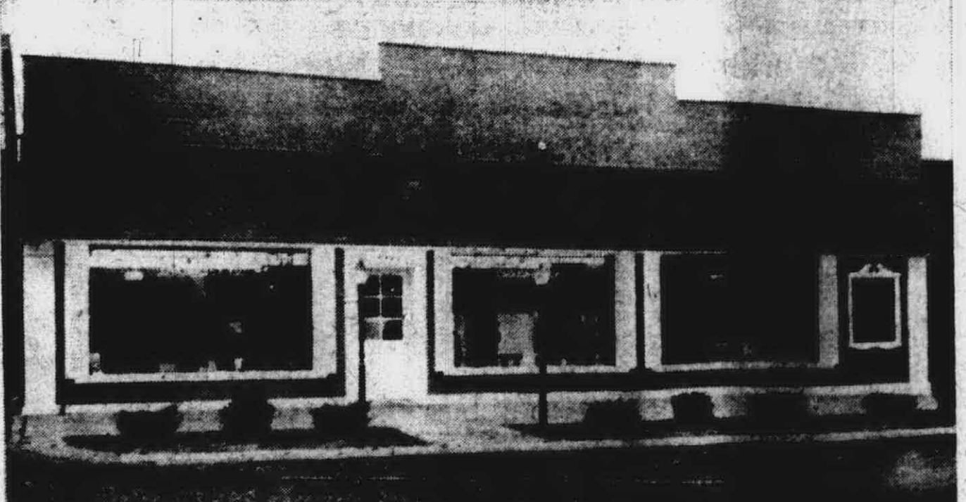
BUILT 46 YEARS ago, this Starkweather Ave. building was first used as a service station, later as a garage and recently as a mover's warehouse.
