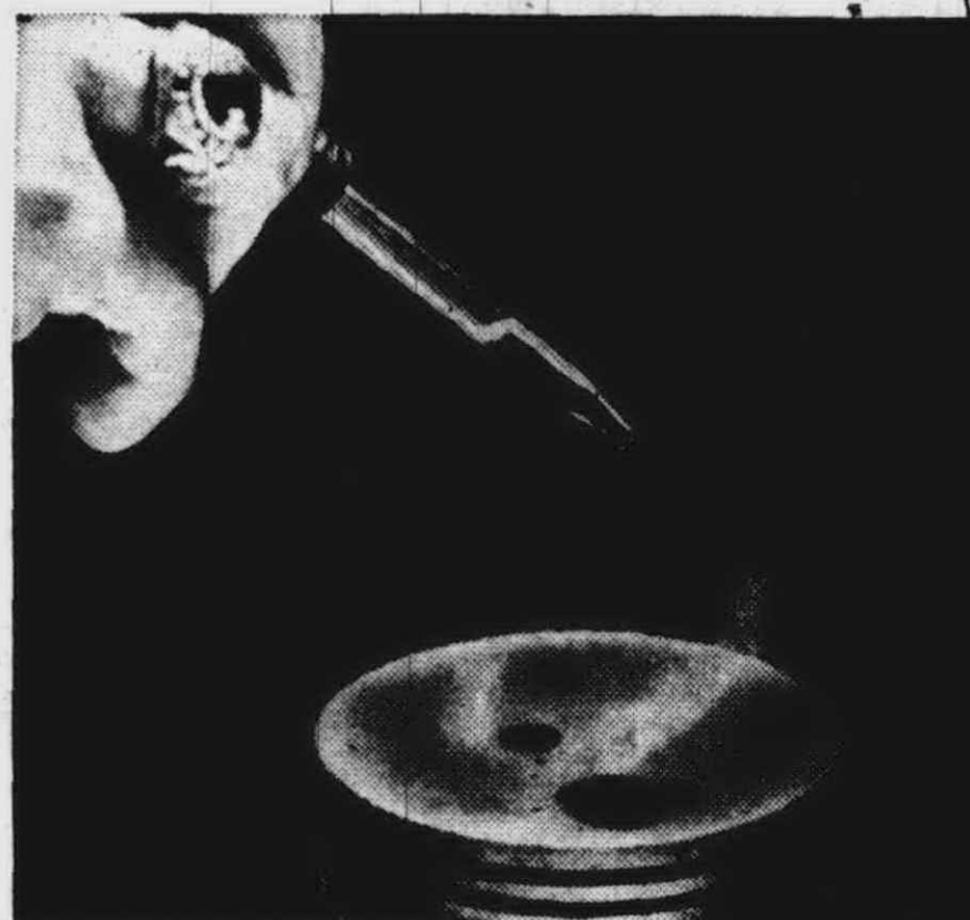
Ordinary oils can create their own metallic ash. Above you see what happens when a conventional multi-grade oil is dropped on this electrically heated piston device. These dark spots contain additive ash. When this ash builds up in your engine, it's bad news.
