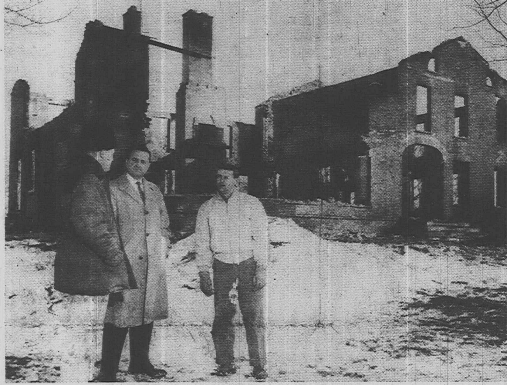
AUTHORS of Civil War books have often described gutted plantation homes of the deep South. Such a picture is brought to mind as one looks at the 17-room home at Napier and Warren Roads that was destroyed by fire Sunday night. The home, built in 1837, was being remodeled. From left are David Dahline, one of the home's owners, Orville Rouse of the State Police Fire Division, and Canton Fire Chief Fred Korte, Jr.
