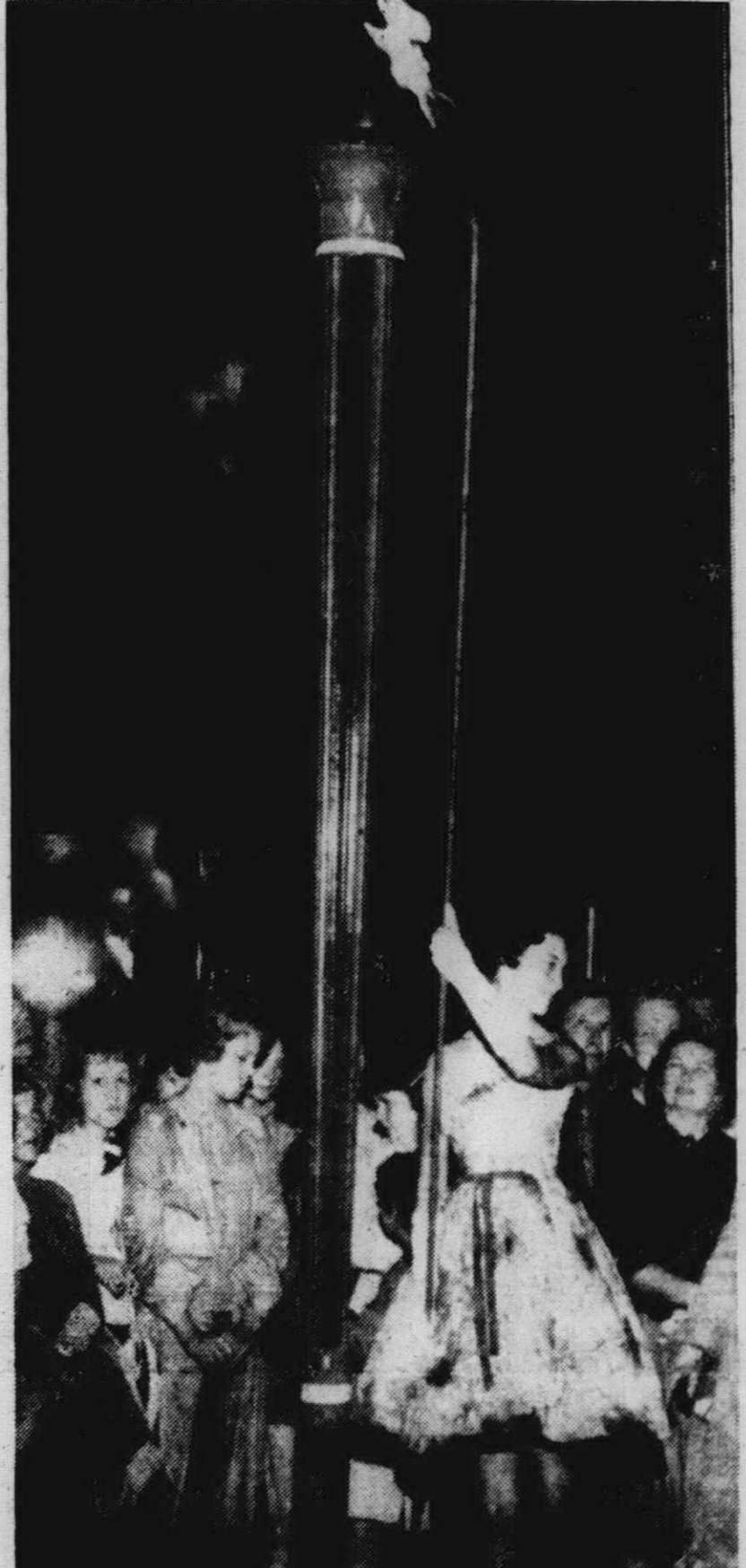
LIGHTING THE torch to officially open the 1960 Plymouth Community Fund campaign last Friday night was Miss Sue Cooper, daughter of Mr. and Mrs. J. E. Cooper, 1375 West Ann Arbor Trail. The torch will burn in Kellogg Park throughout the drive.
